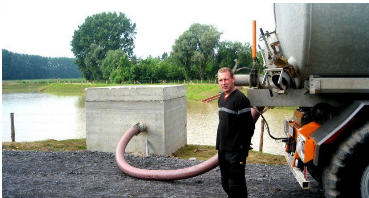
Figuur 71: Aftappunt thv bufferbekken in Vlamertinge (bron: www.focus-wtv.be )
